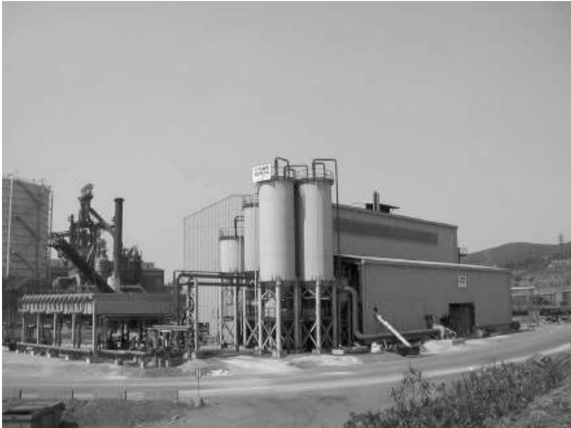
Picture 1 Overall view of the demonstration plant in Piombino
